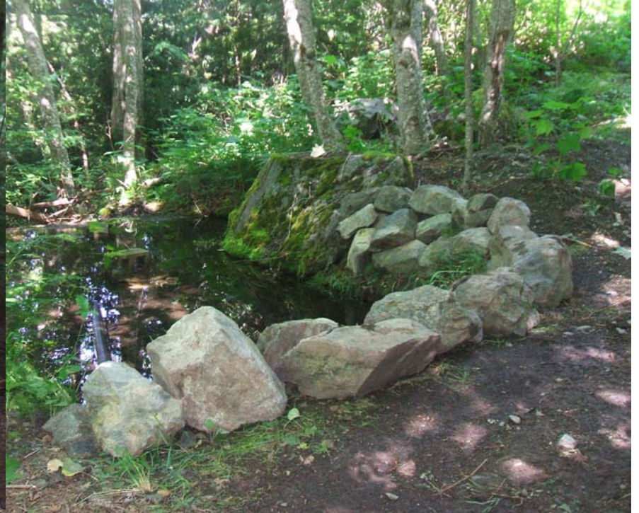
A Rock Embankment was built around the Drinking Water Collection Pond
